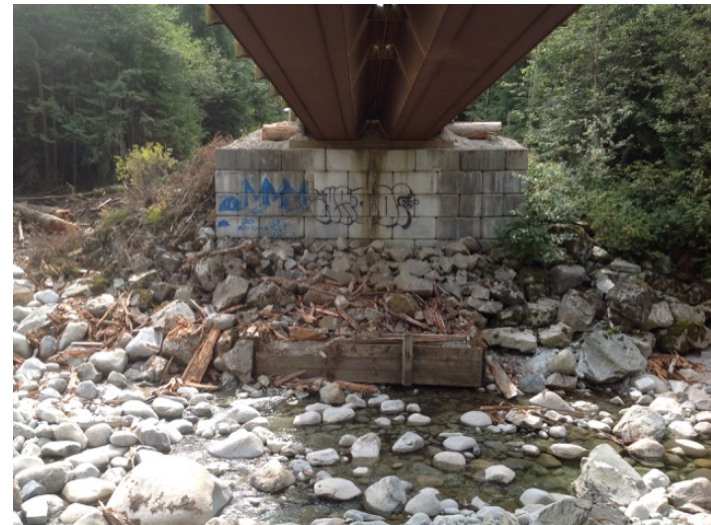
Left Bank Abutment when facing downstream
