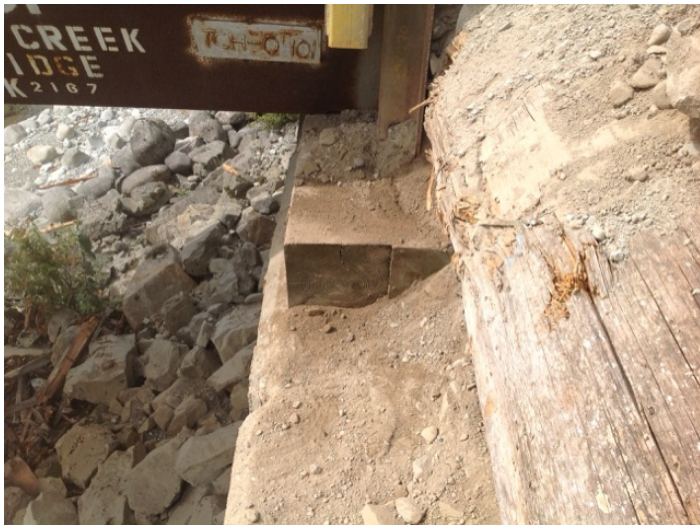
new treated timber sills
