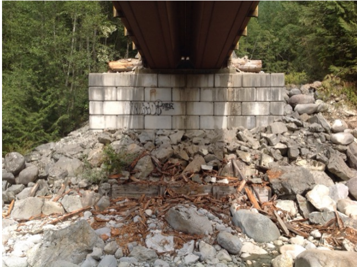
Right Bank Abutment when facing downstream
